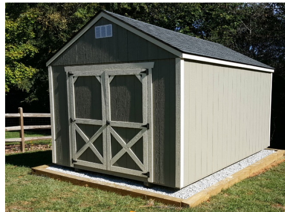
Shed on Gravel Base with 12-inch gravel border.
