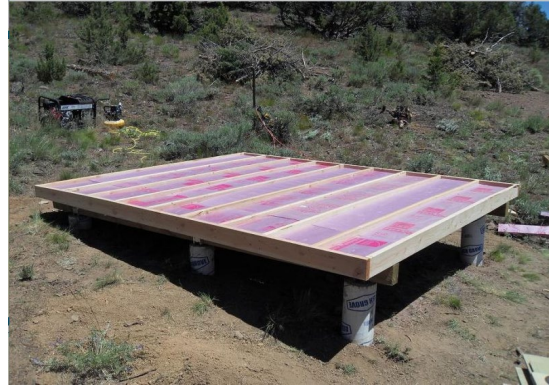
Example of a shed floor on Pier Footings
